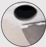
Trimless installation in plaster board
